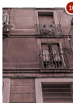
C. Pedreres Barcelona Sants-Montjuïc district
